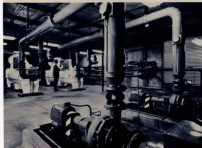
Chiller Plant – two 150 ton units
